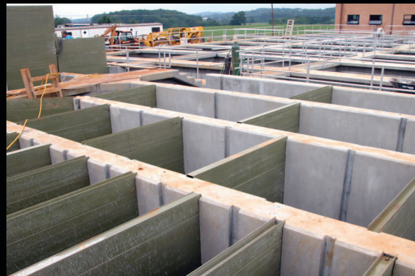
WWTP Baffle Panels | Greeneville, TN
