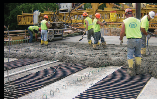
Stay-In-Place Concrete Forms | Black River Falls, WI
