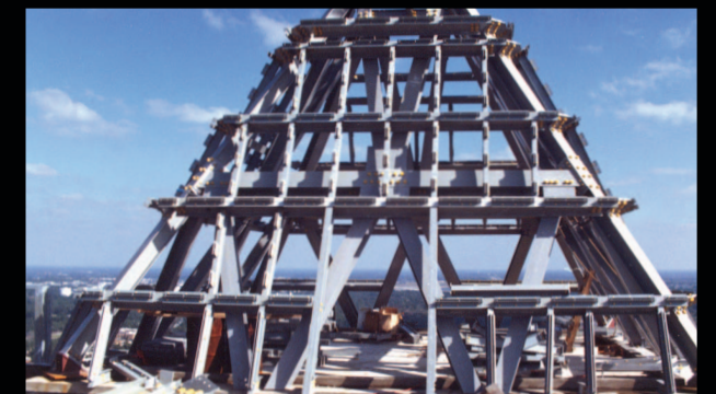
RF Transparent Rooftop Structure | Orlando, FL
